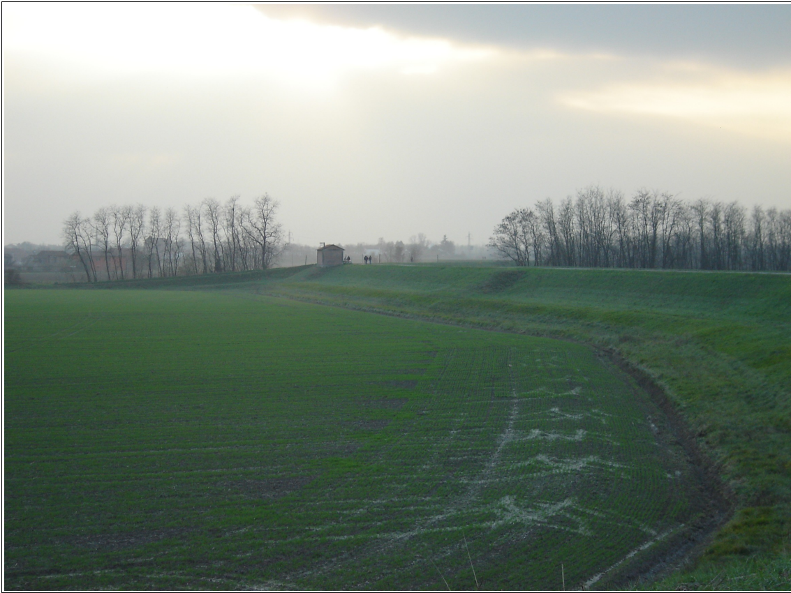
Figure 1: The elevated road/levee across the river Po plain (November 2009)
